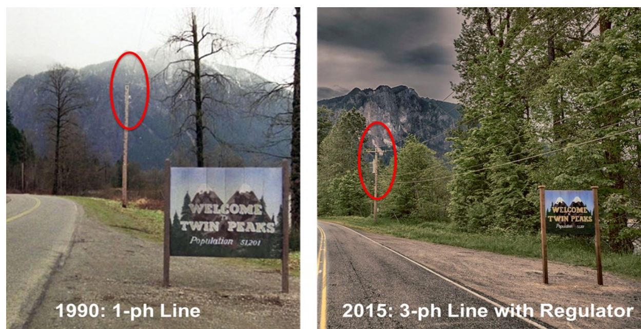
Figure 9: Comparison of historical photos of a distribution line running along Reinig Road, Snoqualmie, WA. Between 1990 and 2015, the distribution line was upgraded to a 3-phase line with additional volt-var control equipment.
